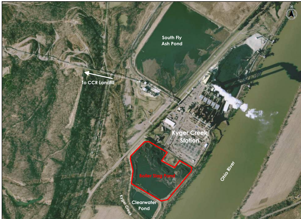
Figure 1. Aerial View of Kyger Creek Station
