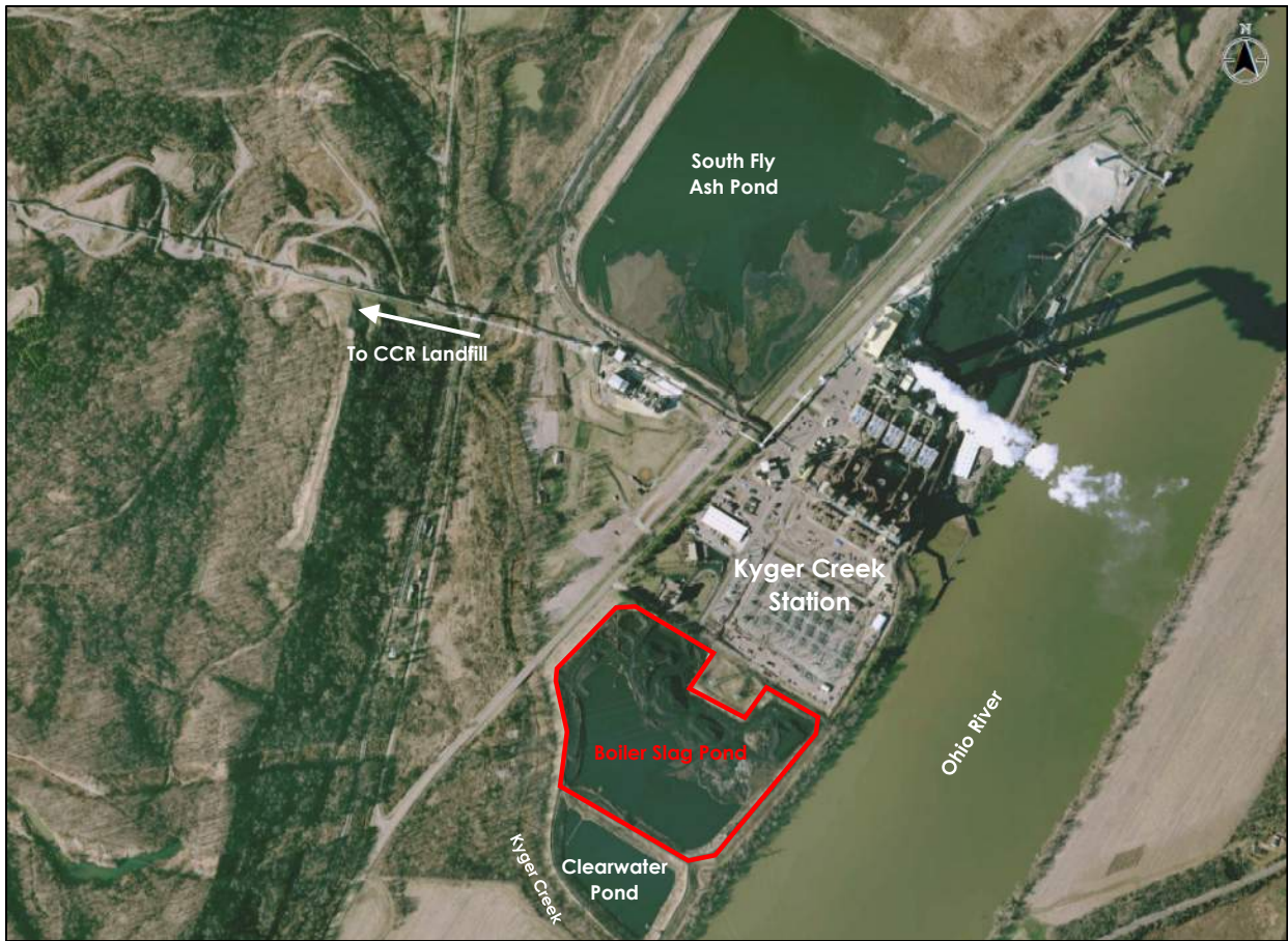
Figure 1. Aerial View of Kyger Creek Station
